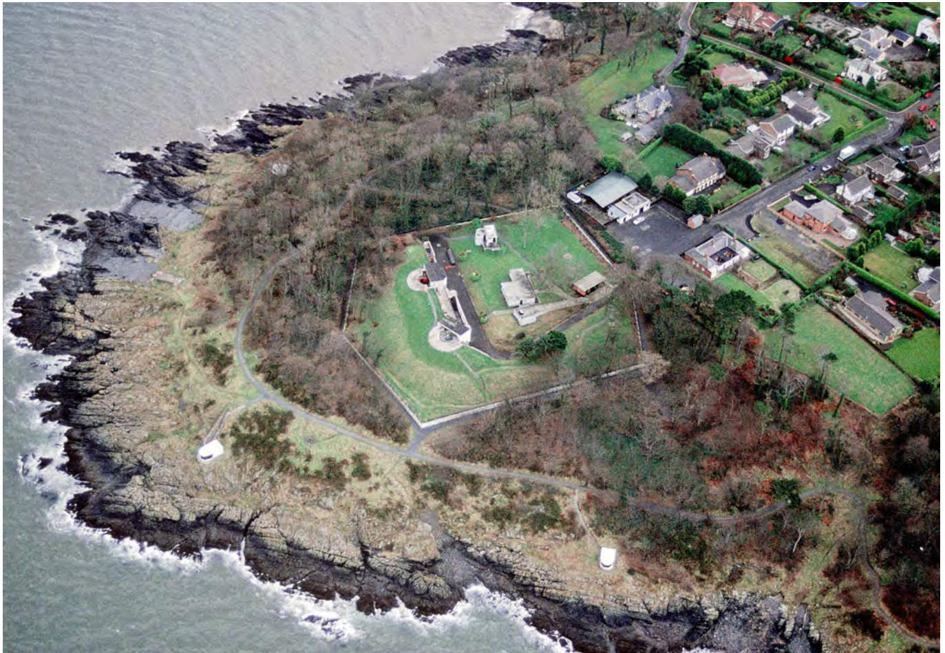
Grey Point Fort's pentagonal form and promontory location are clearly seen from above.
